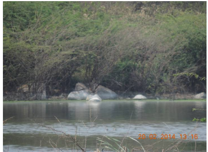
Fig.1.21: A photographic view of the Premajipet Tank (L10).
